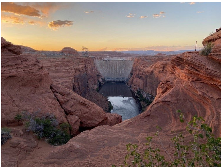
Figure 3: Glen Canyon Dam
